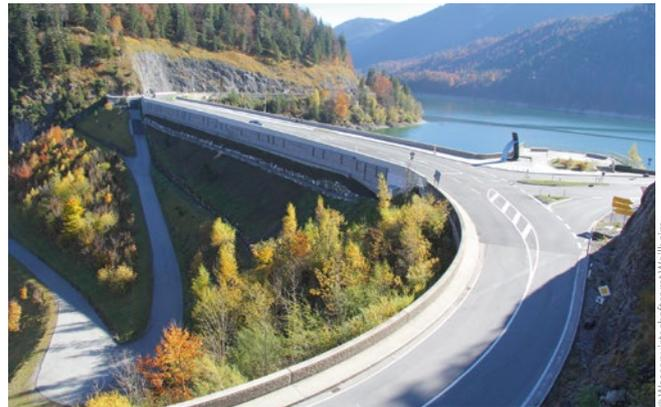
Figure 10: The new B 307 over the widened dam crest in autumn 2015
