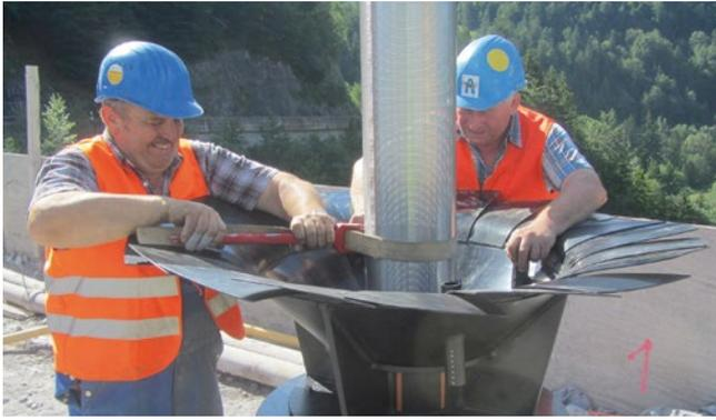
**Figure 8:** Preparations to install the drainage filter (slotted pipes and sump pipe)
