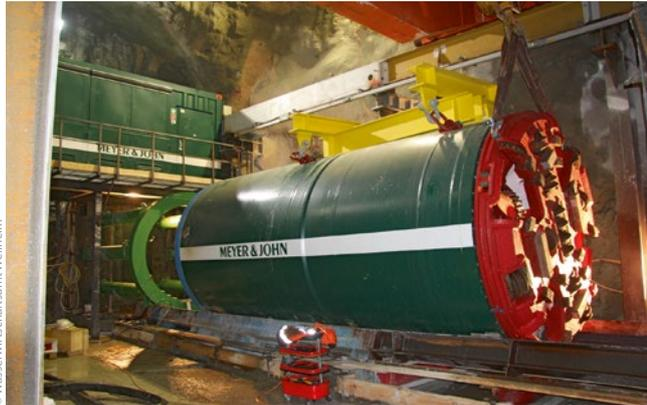
**Figure 6:** Installation of the TBM on the cradle; behind it the press station with six hydraulic cylinders for 2,500 t thrust and above it the driving control station
