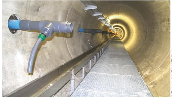
**Figure 9:** View of the inspection gallery with the seepage collection system and interior fitting
