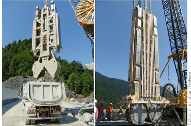
**Figure 5:** The Bauer Spezialtiefbau diaphragm wall grab and hydromill cutter in operation
