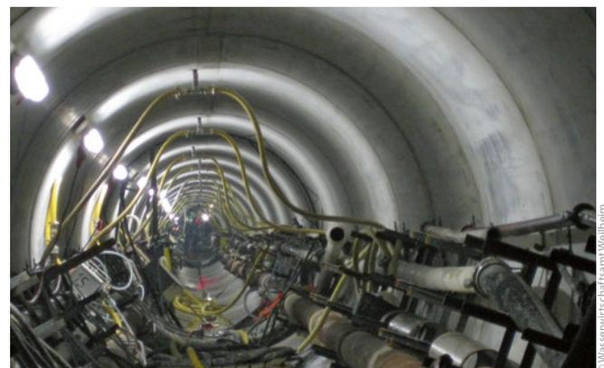
**Figure 7:** Tunnelling, laser, transport and supply lines, bentonite grouting to reduce surface friction takes place using the yellow grouting line
